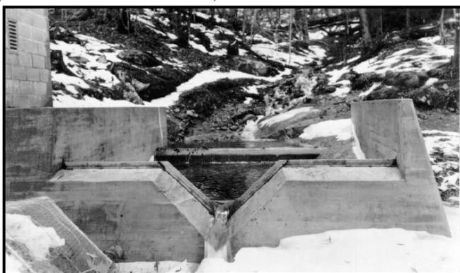
**Figure 1:** Compound notch, suppressed rectangular with  $90^\circ$  triangular notch
